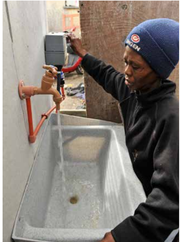
Basic services include a refuse bin per yard, a wash trough and tap attached to a pre-cast flush toilet, as well as electricity connections for up to three structures.
