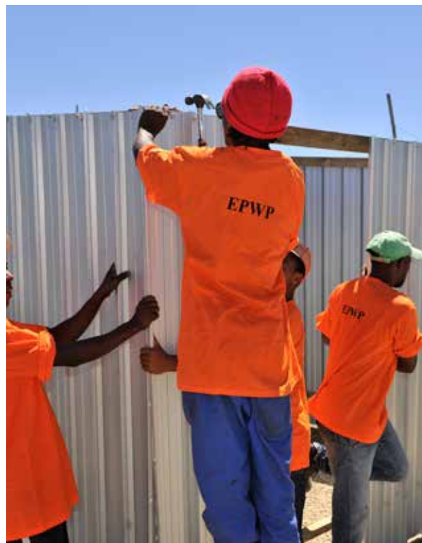
EPWP workers assembling a dwelling with an enhanced emergency housing kit.
