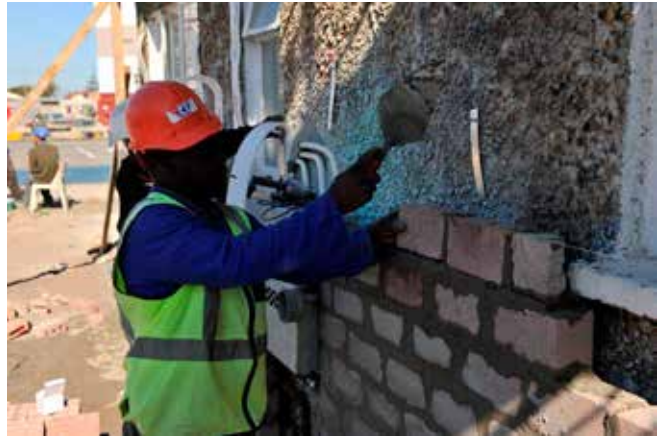
Brick skins being applied over existing old exterior.
