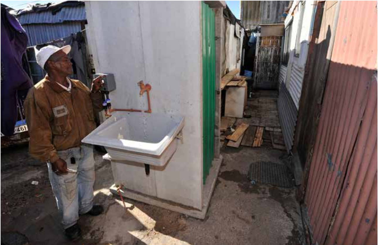
Precast structures containing a flush toilet, a tap and wash trough for use by families living in backyards of Council rental stock.
