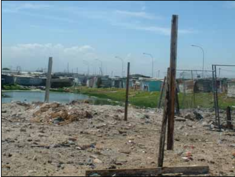
Picture 5: Encroachment of informal settlement into a storm water detention area
