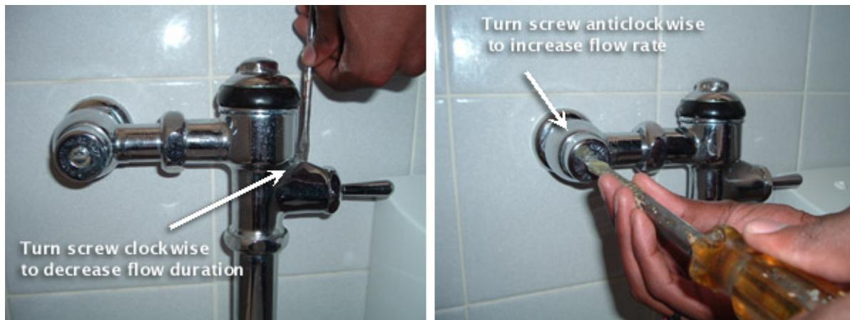
To reduce the flush duration, turn the screw above the handle clockwise. To increase the flush intensity, turn the screw on the bend exiting from the wall anticlockwise to open the inlet valve. If these settings result in water splattering on the toilet seat then the intensity of the flush will have to be reduced and the duration may need to be increased. If the flush remains unsatisfactory then a new set of rubber seals may need to be installed by a suitably experienced person.
