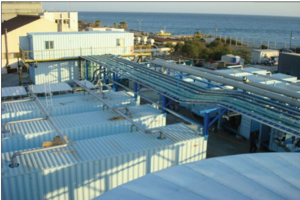
Figure 3 – 20 MLD Containerized SWRO Desalination Plant in Cyprus
