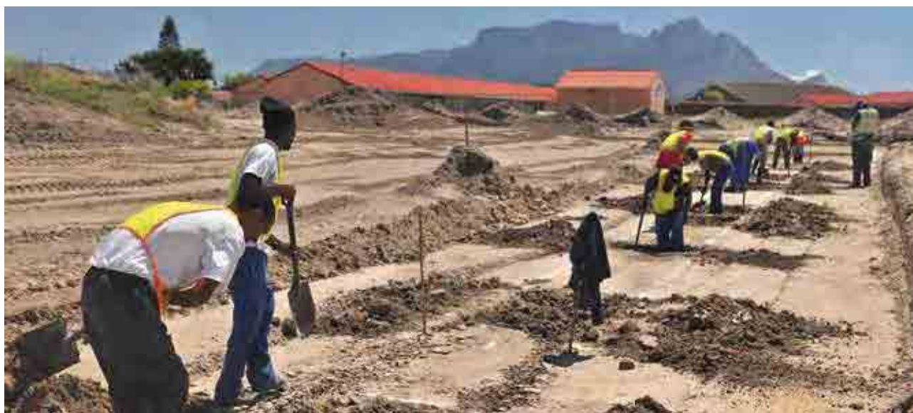
Preparation for a new housing development.
