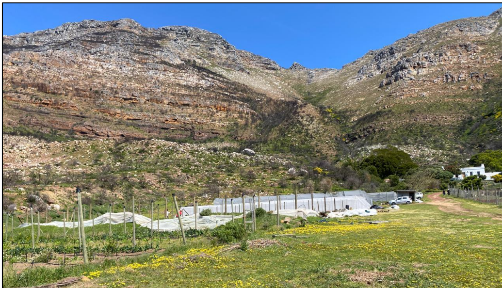
Figure 7. Repairs are underway on the vegetable tunnels at Rocklands Farm.
