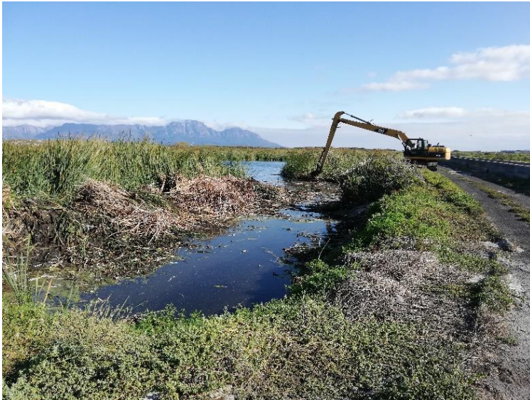
Figure 51: Bulrush ( Typha capensis ) clearing activities with the assistance of an excavator within the FBNR: Strandfontein section to improve bird habitat
