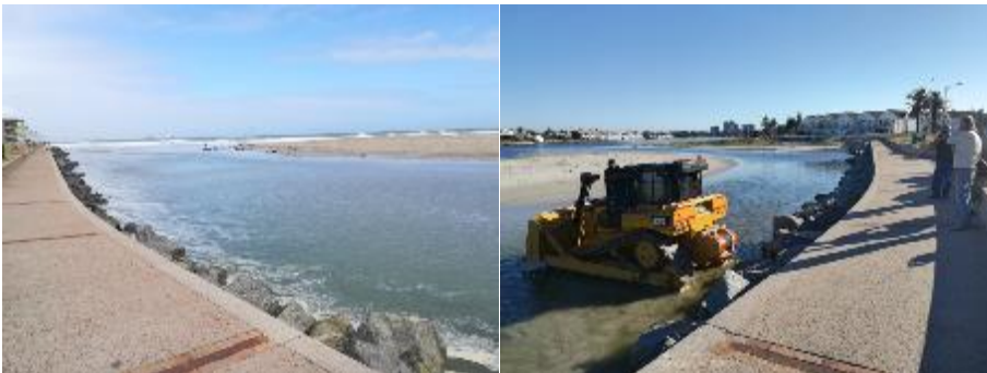
Figure 47: Natural breaching of the Milnerton Lagoon estuary mouth and the bulldozer used for artificial breaching work.
