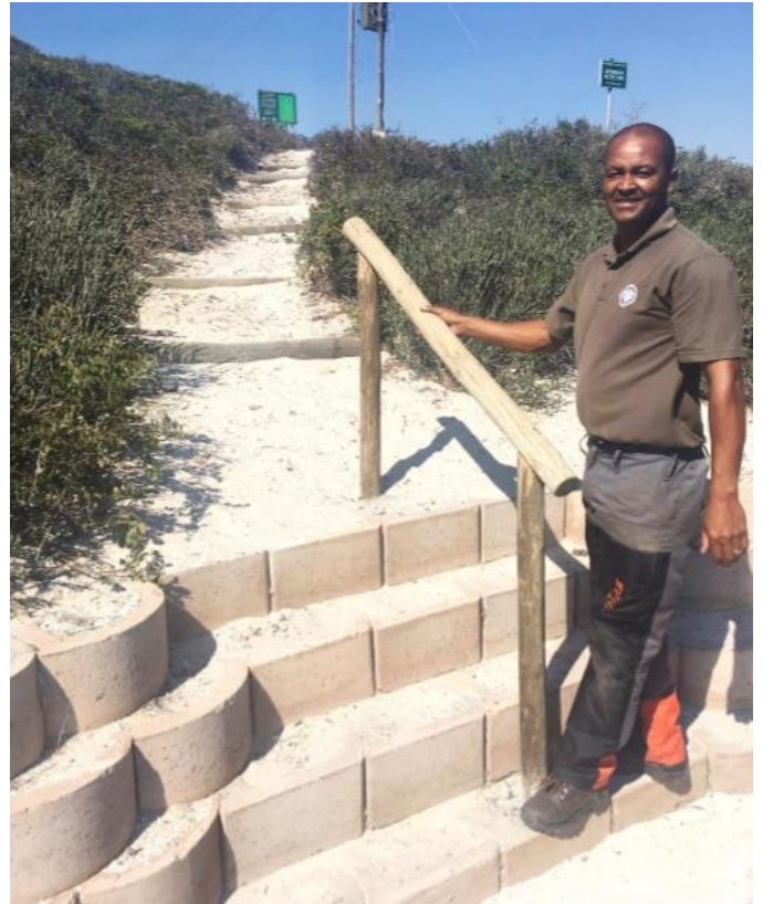
Figure 71: Erosion control measures and a hand-railing installed at the start of the Coastal Hiking Trail.
