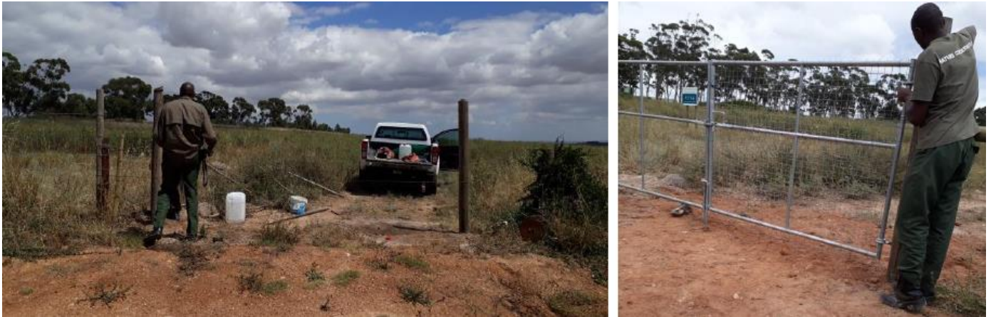
Figure 144: Erection of gate at Joostenbergskloof main entrance.
