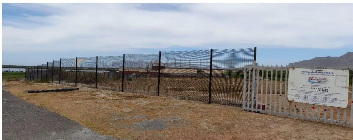
Figure 167: New fencing at the Strandfontein section of False Bay Nature Reserve.
