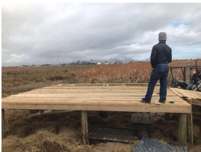
Figure 165: The completed deck at the Friends of Rietvlei Bird Hide.
