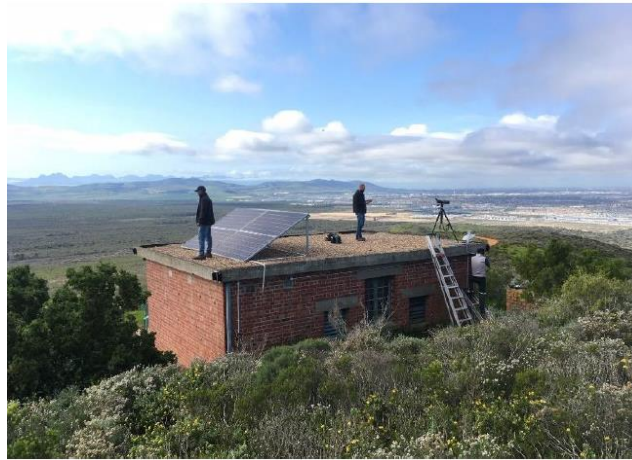
Figure 106: Installation of part of the CCTV system at Blaauwberg Hill.
