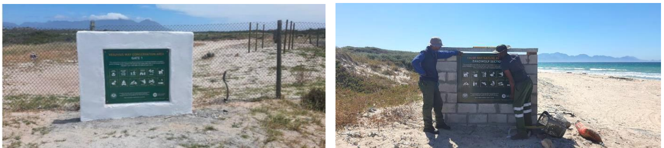
Figure 118: Signage installed and painted at entrance of VEWS (left) and construction of signage wall at Nautilus beachfront (right).
