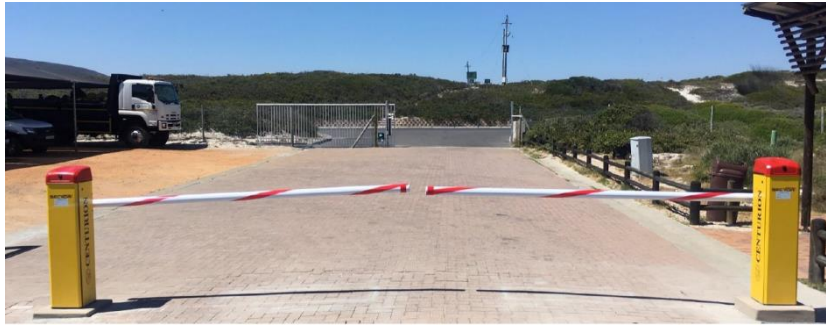
Figure 111: Reinstated access control booms and electrified gate at Eerste Steen Resort.
