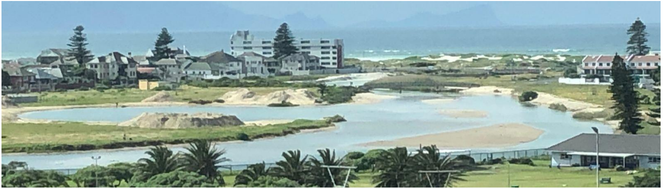
Figure 48: Sand dredged out of Zandvlei can be seen on the shoreline as it dewater before transport
