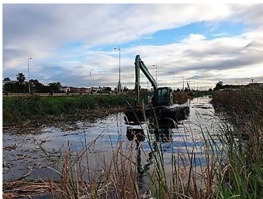
Figure 45: The amphibious excavator clearing material in Bayside Canal.
