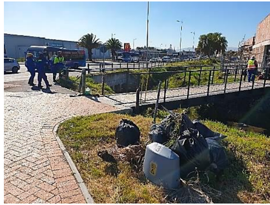
Figure 47: EPWP contractor cleaning the stormwater outfalls and canals.
