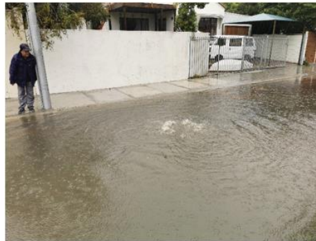
Figure 40: Sewage spills do not always occur in the nature reserves. Here sewage is overflowing from Rutter Road, Lakeside, where it will flow into Zandvlei Nature Reserve.
