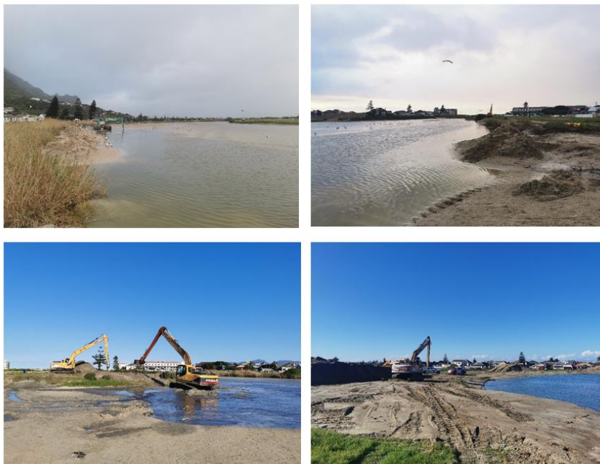
Figure 49: Sand sediment being removed from the Zandvlei Estuary mouth
