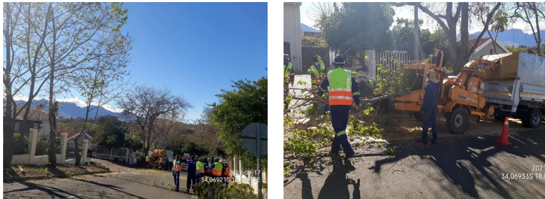
Figure 74: Contractors removing PSHB infested trees, Somerset West.
