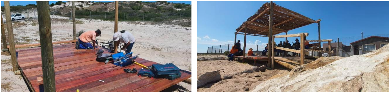
Figure 117: Construction of outdoor classroom at VEWS (left) and its completion (right).
