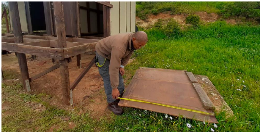
Figure 112: Replacing the old decking floor at the toilet block at Blaauwberg Hill.
