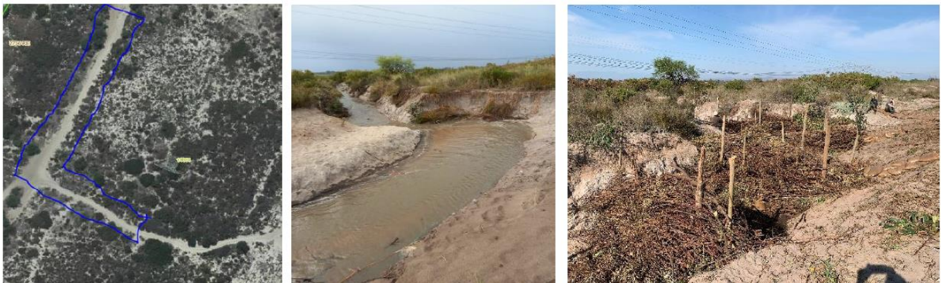
Figure 59: Gabions were constructed as temporary measures until the pipeline was repaired.
