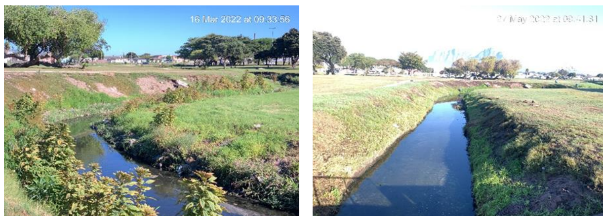
Figure 68: Photographs depicting Vygekraal Reach 3 before and after clearing operations.
