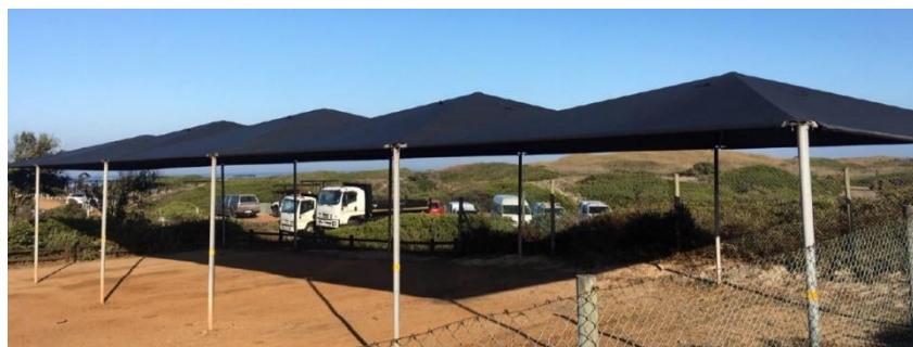
Figure 110: Repaired parking shade port for Council vehicles at the Eerste Steen Resort.
