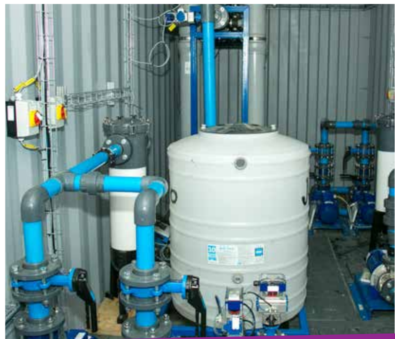
Installation of our reverse osmosis desalination plant
