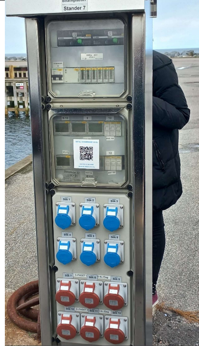
Figure 101: Close-up of the charging station sockets. Note the QR code that provides easy access to the internet to enable charging with user interface of choosing charging times and payment options.
