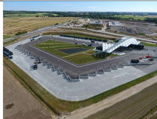
Figure 45: Recycling centre with retention pond in the middle. Skips / bins are stationed on the outer lane (1.5m lower) for ease of access to private vehicles (throwing waste down in the containers instead of up and over a high edge). 24
