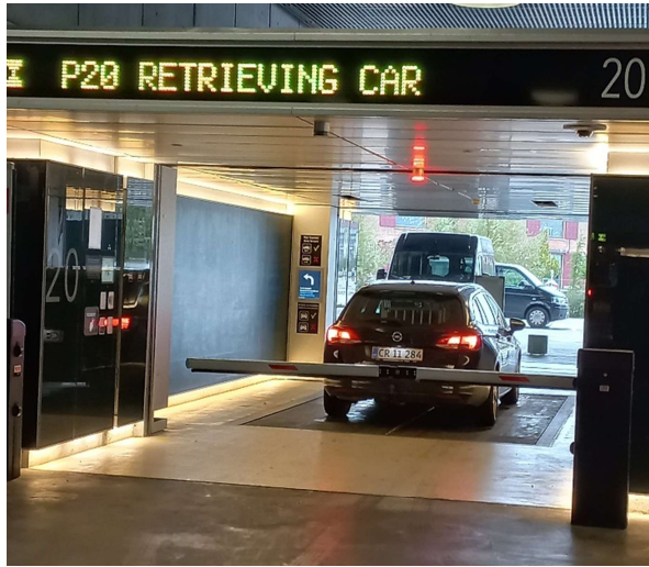
Figure 124: The automatic car park at Dokk1 City library. Here a vehicle is retrieved from elevator cabin 20.
