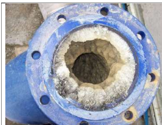
Figure 33: Struvite build-up in WWTP pipes.
