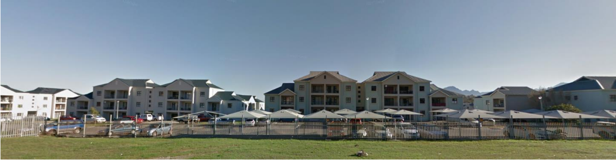
Figure 22 Seascope Mews apartments along Sir Lowry's Pass road (Google Earth, 2019)
