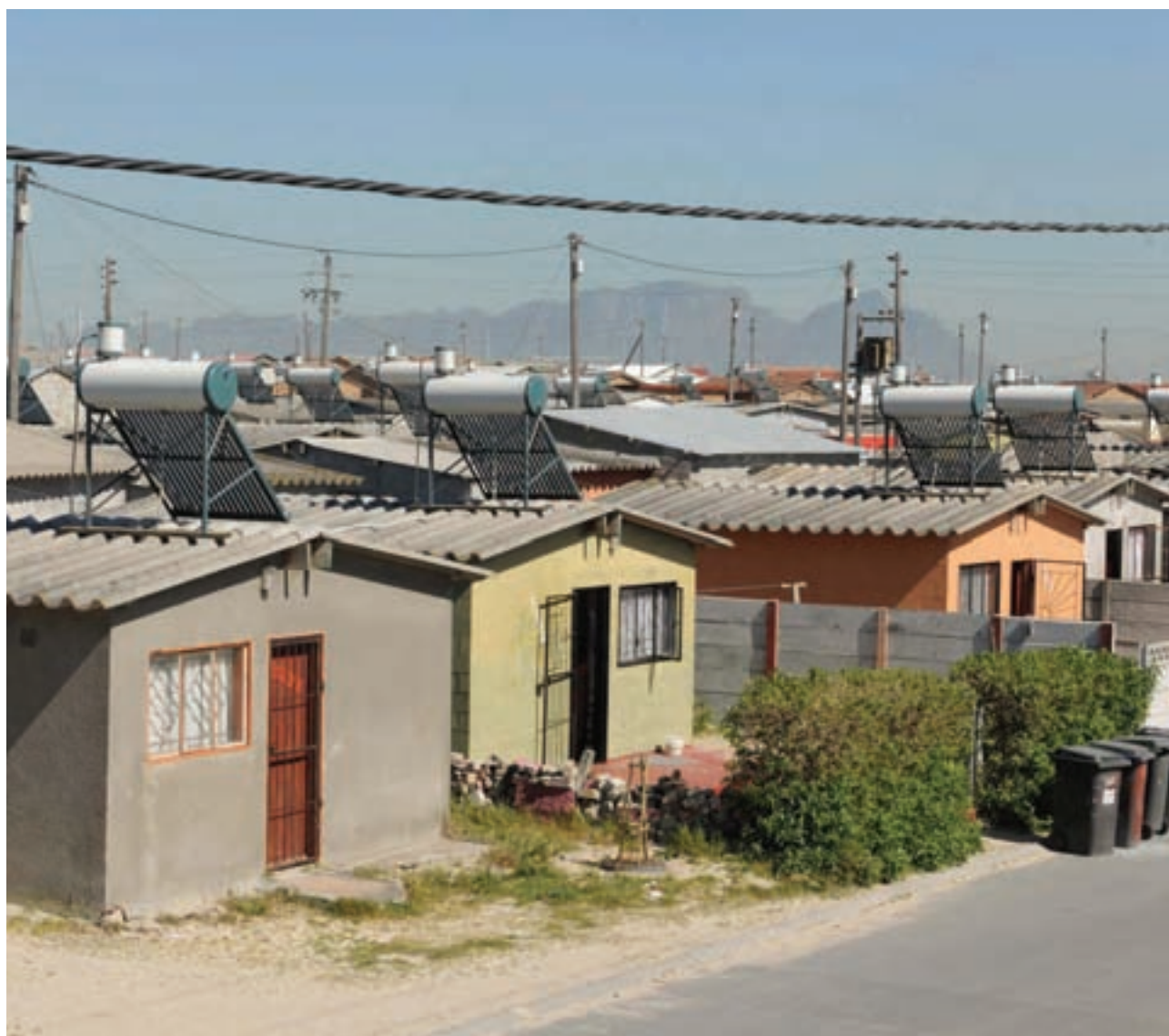
The pioneering Kuyasa housing project provided over 2 000 households with energy-efficient solar water heaters, lighting and ceilings
