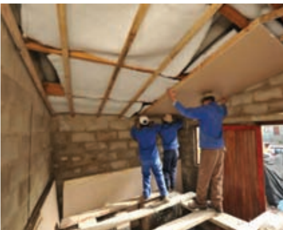
In Mamre several houses were retrofitted with insulated ceilings
