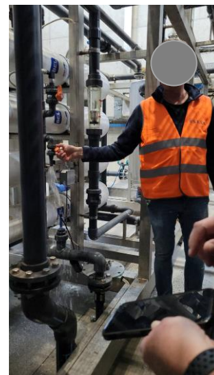
Plate 31: UF treated leachate (permeate)
