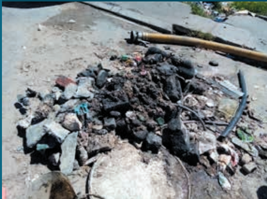
FIGURE 22: BUILDING MATERIAL REMOVED FROM SEWER INFRASTRUCTURE
