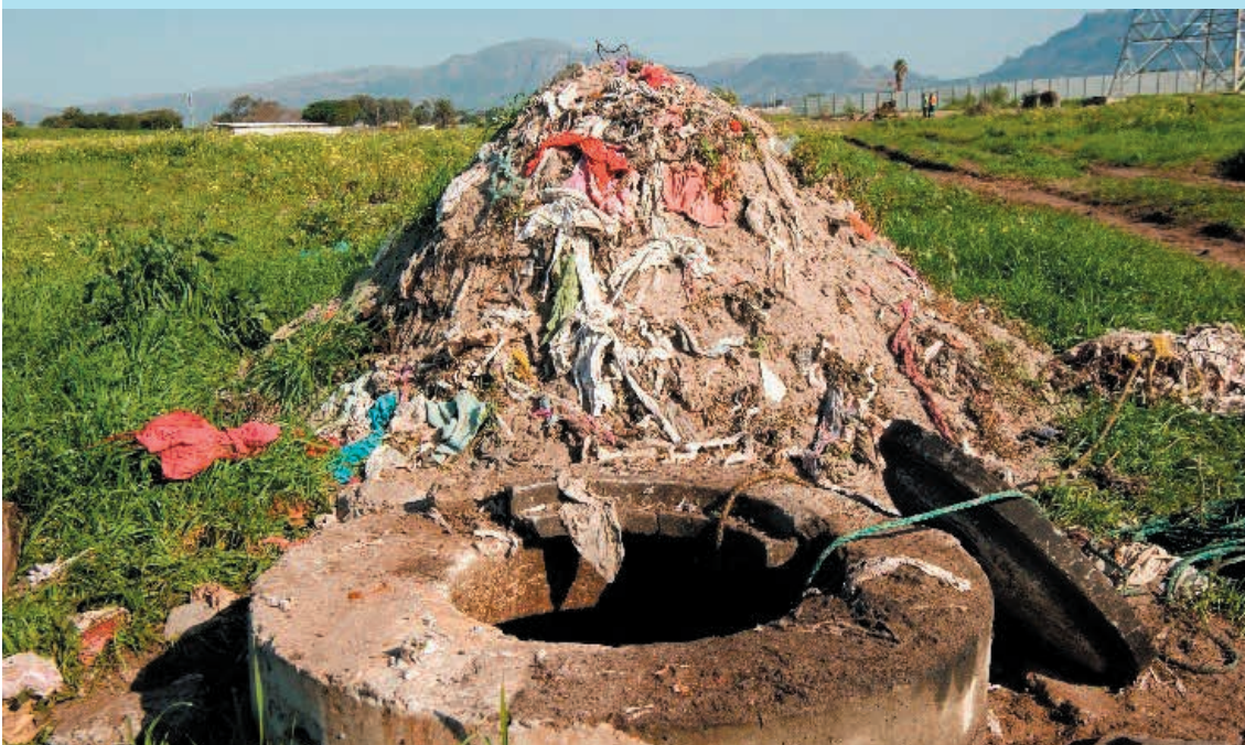
FIGURE 1: FOREIGN MATERIALS REMOVED FROM THE CITY'S SEWER SYSTEM
