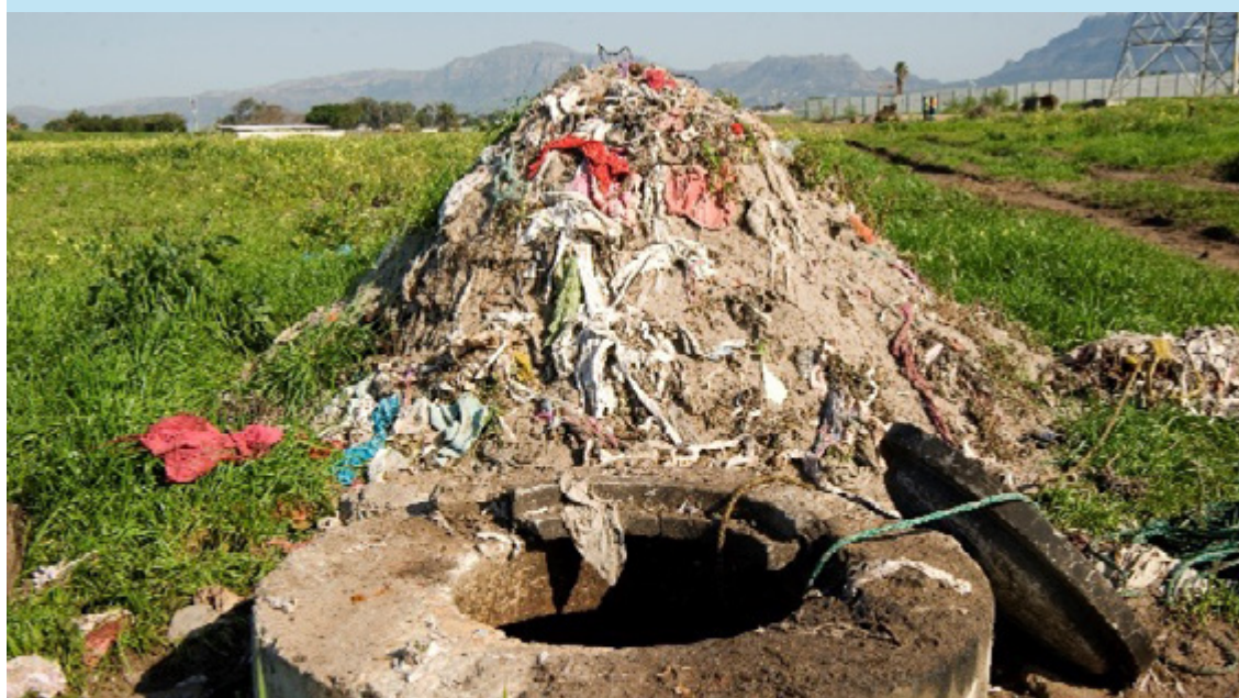
FIGURE 1: FOREIGN MATERIALS REMOVED FROM THE CITY'S SEWER SYSTEM
