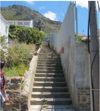
15. Concrete finish on top of brick paving is disintegrating on the stairway and in need of repair.
