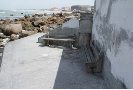
14. Broken benches along the walkway need to be repaired. Wall facing the sea has been painted white to hide graffiti, a more neutral grey colour could be used.
