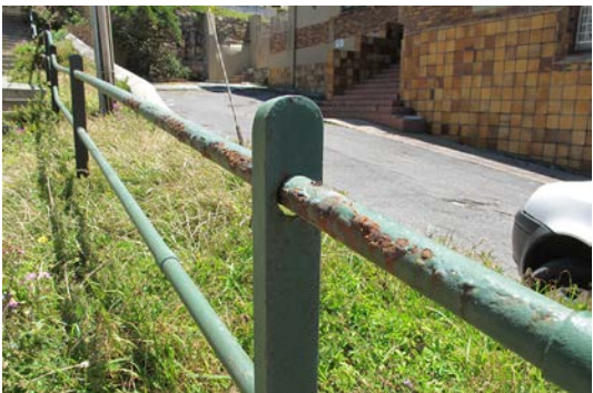
13. Rusted railings need to be replaced.
