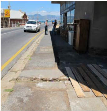
11. Drainage channel in asphalt sidewalk is in need of repair. Water is flooding the pedestrian route. Surrounding asphalt is patchy and in need of repair.
