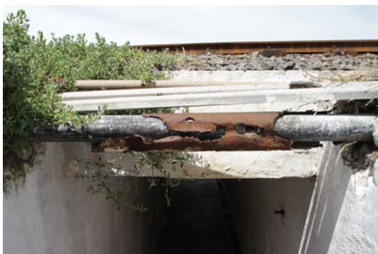
3. Asbestos piping and rusted piping exposed above subway entrance
