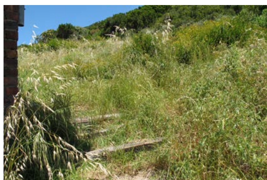
19. Railway sleepers need to be leveled and the footpath should be cleared and clearly demarcated.
