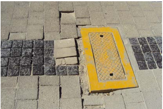
15. Degraded exposed aggregate and cobble paving
