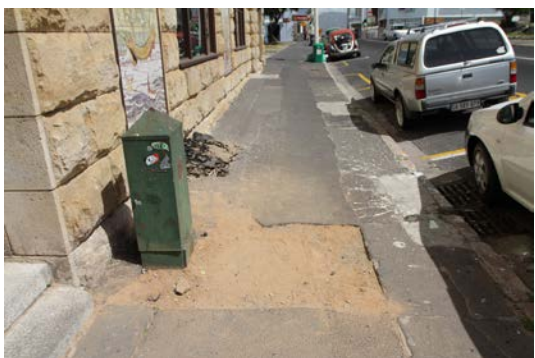
15. Degraded exposed aggregate and cobble paving
