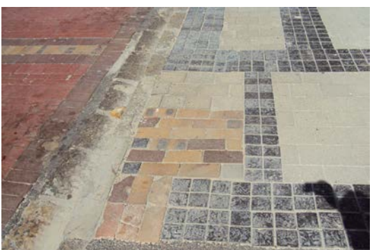
16. Repairs to the sidewalk are made with different paving materials to the original.
