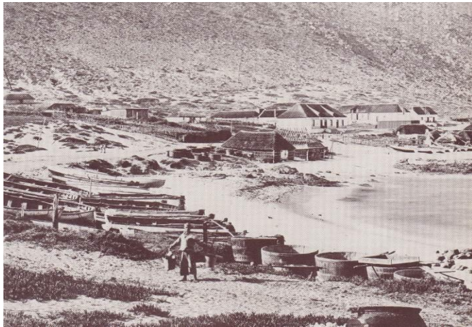
Kalk Bay Fishery beach circa 1875, before the railway line bisected it. Note the whale oil vats in the foreground.
