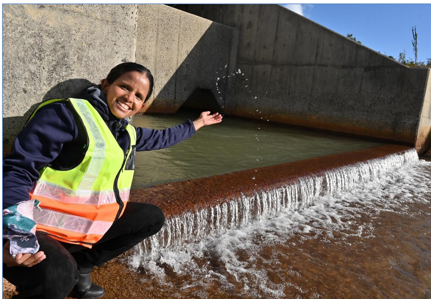
Figure 7 - TMG Steenbras Wellfield First Water – August 2020
