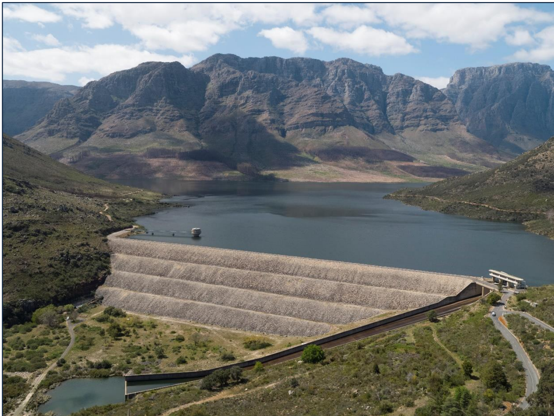
Figure 7- Wemmershoek Dam in October 2020
