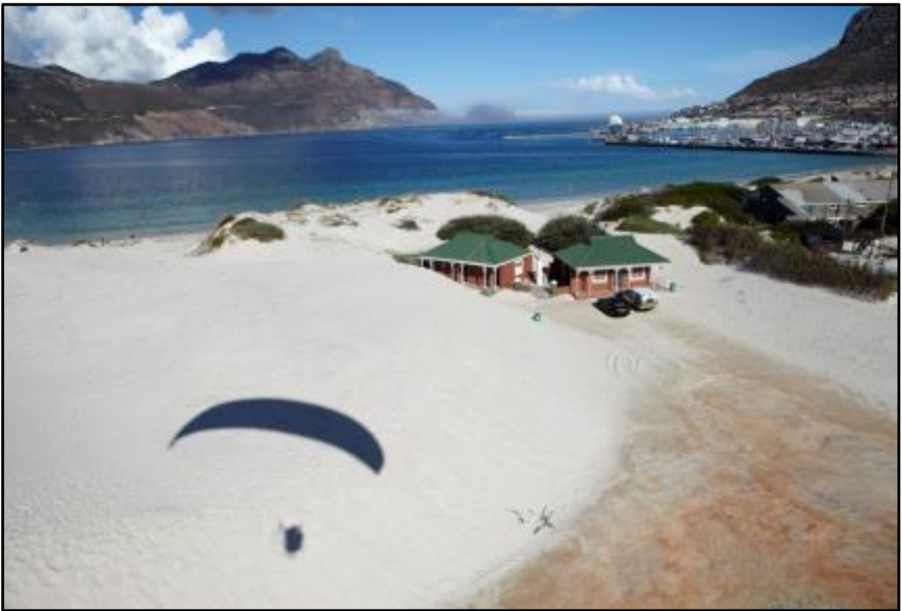
Figure 3: mobile dune systems pose a significant threat to coastal infrastructure if not managed correctly and persistently
