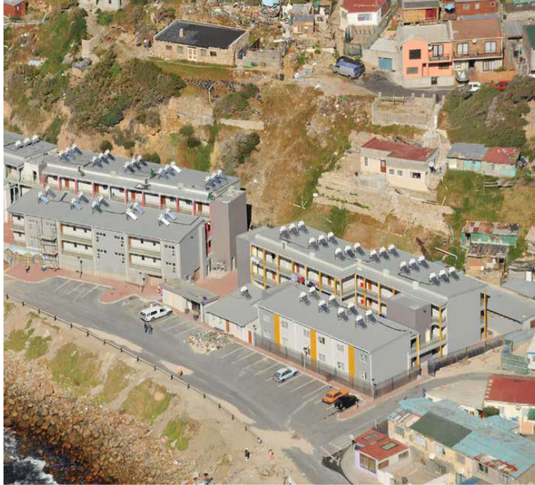
Figure 26: Newly built, non-saleable public rental housing. The Sea Views CRU development in Hangberg consists of 71 rental units
