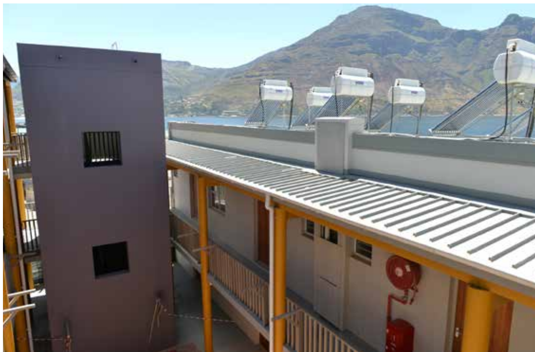
Investing in green technologies when developing housing projects include the installation of solar water heaters.
