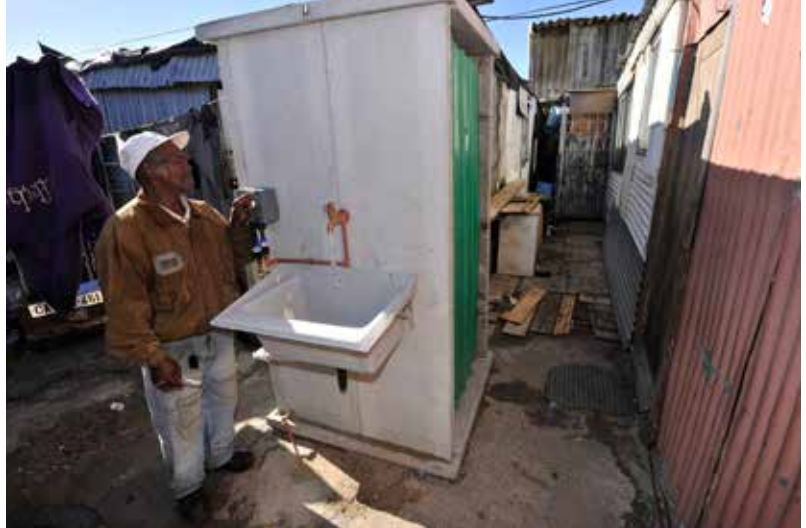
Services to backyarders are provided in the form of a precast structure containing a flush toilet, a tap with a washing trough, electricity connections for up to three structures and a refuse bin per backyard.
