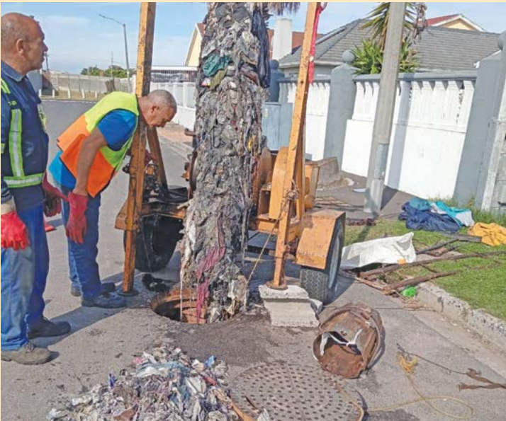
Let it s(t)ink in: Mechanical cleaning of a bulk sewer in Manenberg yielded stacks of rags, nappies, wet wipes and other debris, underscoring the need for behaviour change among Capetonians.
