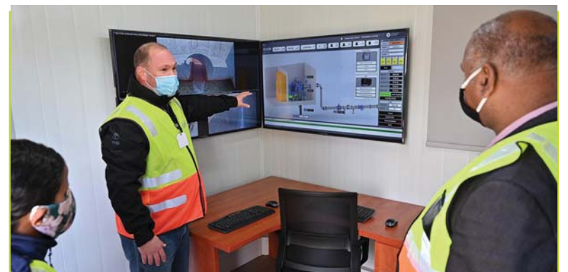
Well, well, well: The new Steenbras groundwater wellfield is controlled remotely.
