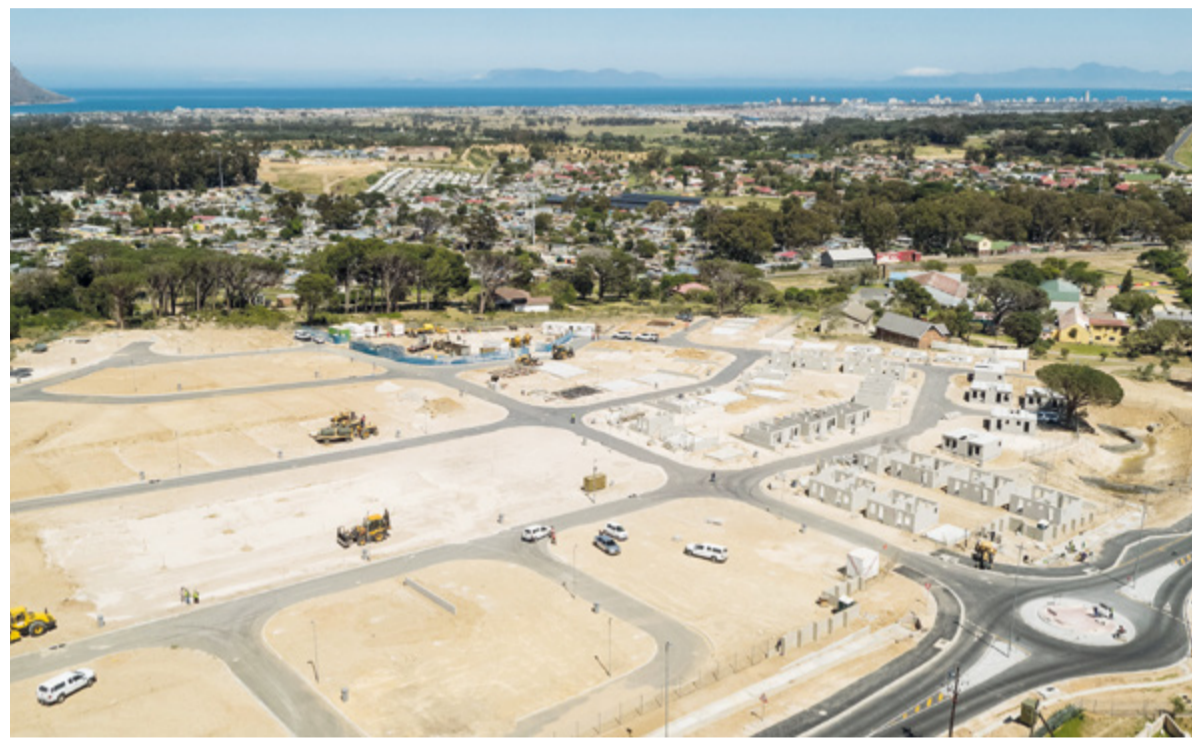
Building a village: Work continues at the City's Sir Lowry's Pass Village housing project. The expenditure will include money for bulk earthworks, internal civil engineering services for the provision of water, sanitation and roads, electricity reticulation and street lighting. The R101 million project will provide 307 housing opportunities – either freestanding or semidetached duplex units – to qualifying beneficiaries.
