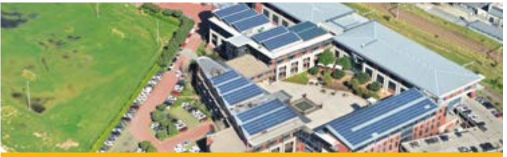
Grid-tied PV system at Black River Park.
