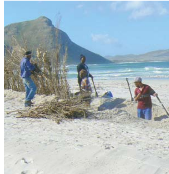
Vegetation is used to trap windblown sand and build dunes.
