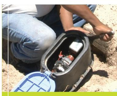
Installation of a water management device (WMD)
