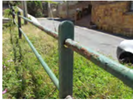
13. Rusted railings need to be replaced.
