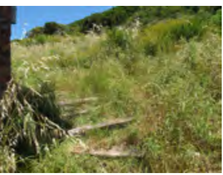
19. Railway sleepers need to be leveled and the footpath should be cleared and clearly demarcated.
