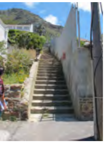
15. Concrete finish on top of brick paving is disintegrating on the stairway and in need of repair.
