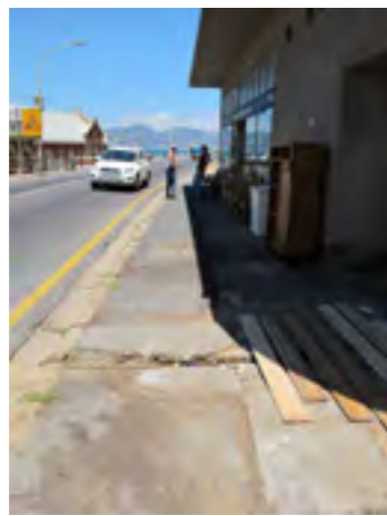
11. Drainage channel in asphalt sidewalk is in need of repair. Water is flooding the pedestrian route. Surrounding asphalt is patchy and in need of repair.
