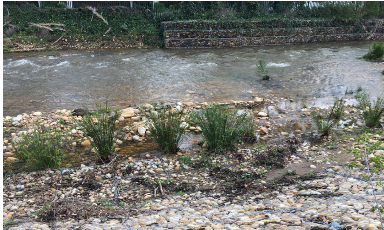
Figure 13: Example of gabion baskets (far bank), and gabion mattresses (near bank), along with riparian vegetation planting along mattress edge.
