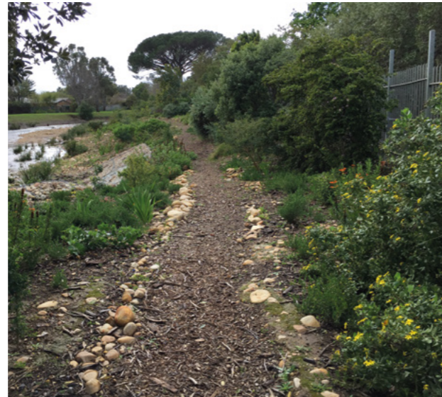
Figure 10: Pervious walkway along the Lourens River. Note landscaping with suitable plant species and appropriate palisade-type fence on the property boundary.
