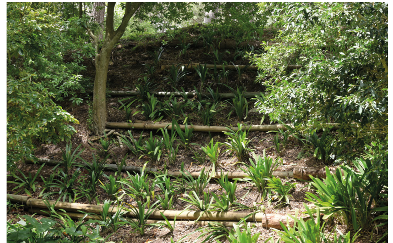
Figure 29: Bank stabilisation using horizontally secured logs between which suitable species are planted.
