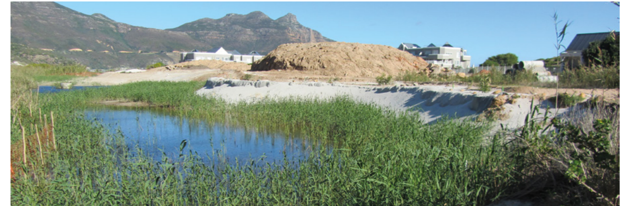
Figure 8: Inappropriate and illegal construction activities within the floodplain.
