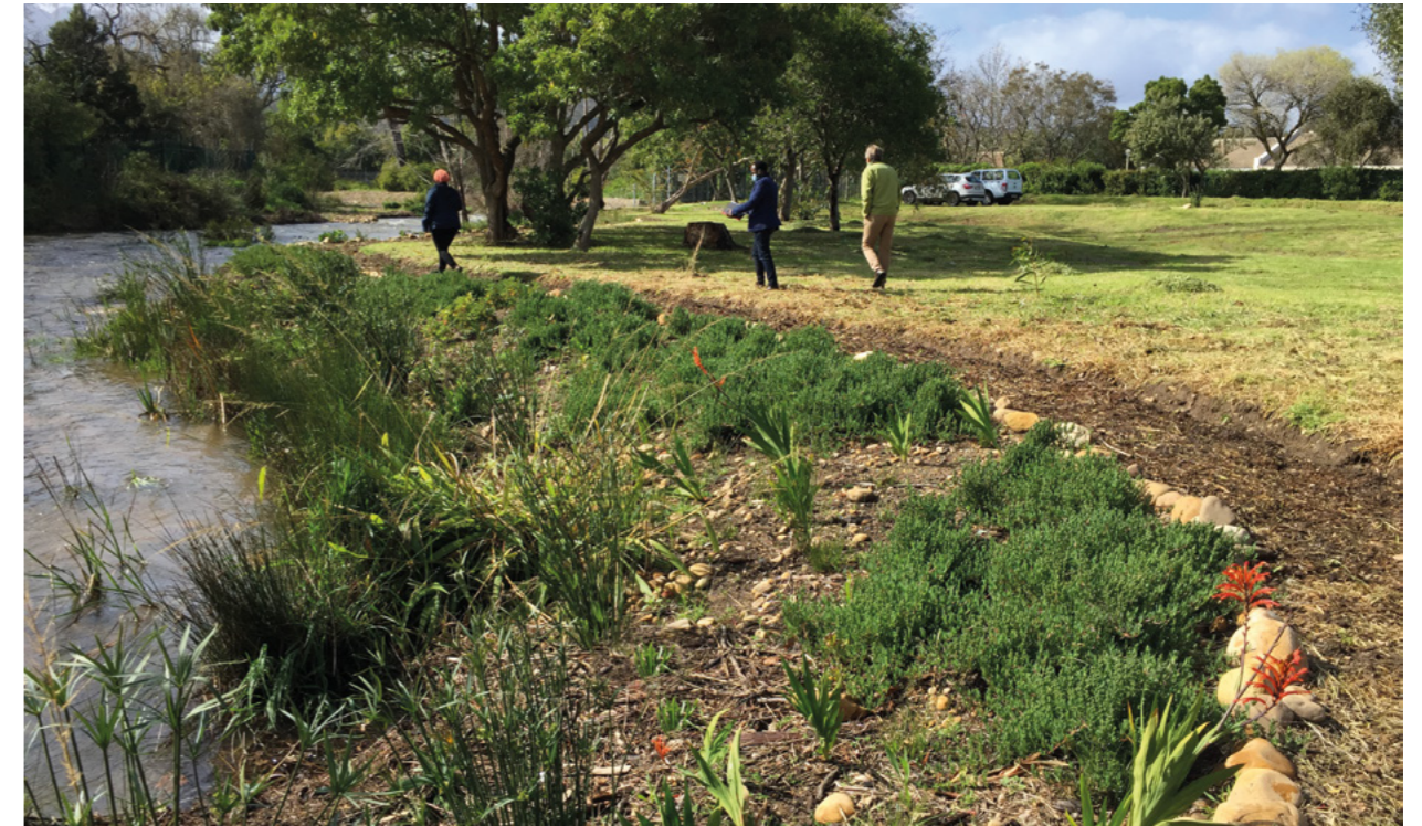
Figure 14: Example of a river bank where riparian planting is being used for stabilisation.
