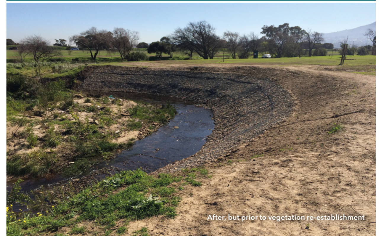
Figure 12: Eroded river bank, which has been shaped and stabilised using gabion mattresses.
