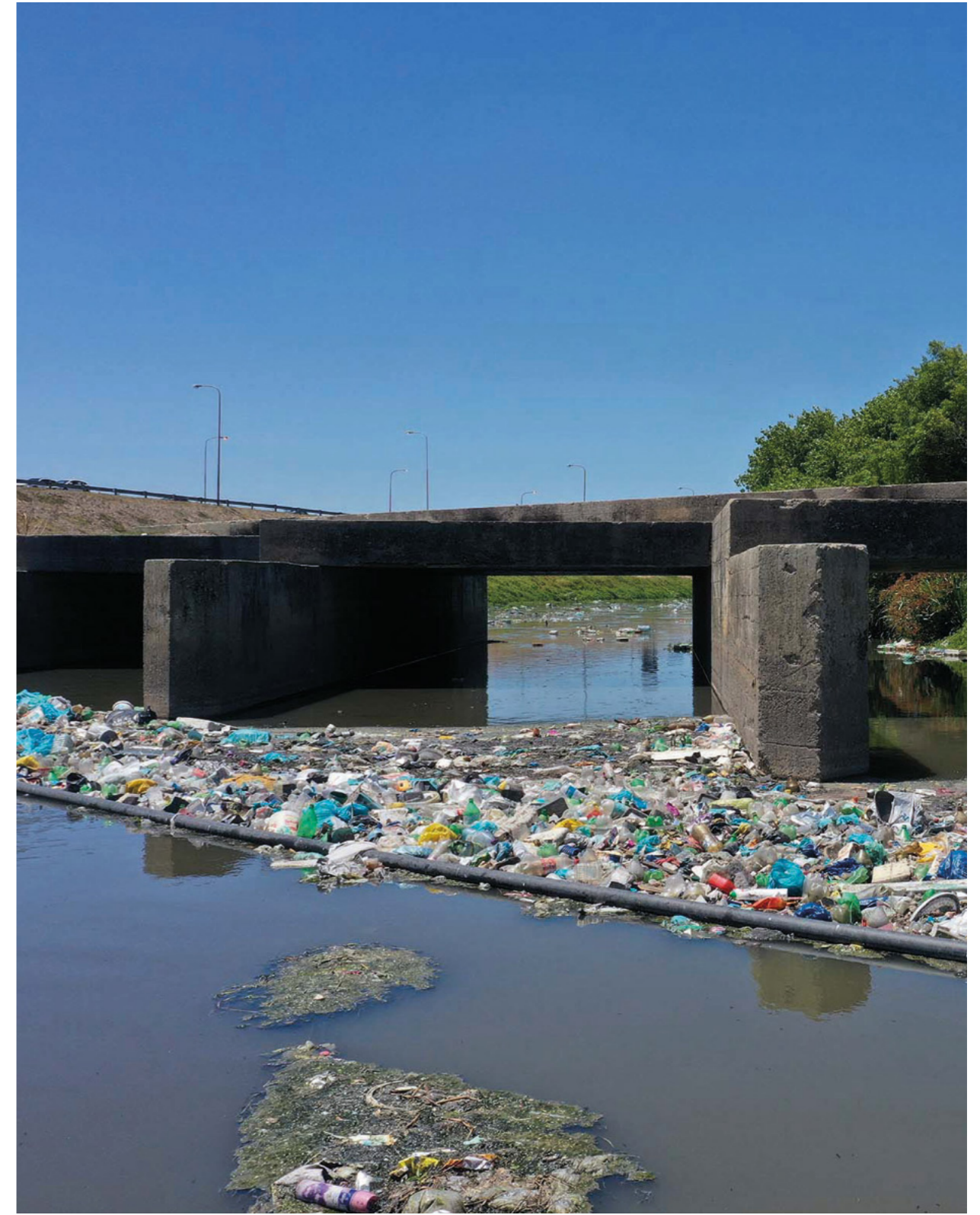
Figure 18: Solid waste caught by a litter boom.
