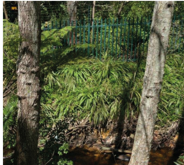
Figure 9: Property adjacent to a watercourse with appropriate permeable palisade-type fencing.
