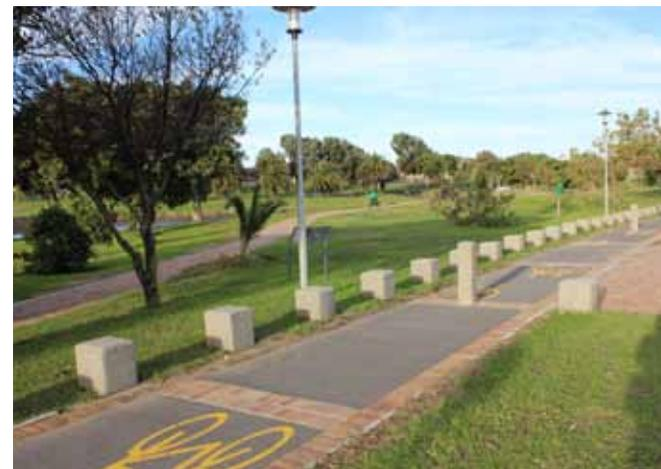
LOW AND HEAVY BOLLARDS CAN BE USED TO PREVENT VEHICULAR ACCESS TO OPEN SPACES
