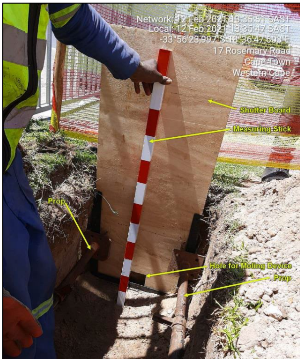
Figure 5-1: Pit for moling process
