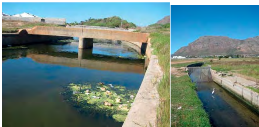
Fig. 11 (a) Accumulated litter in the Sand Canal just above the point of discharge into Zandvlei; and (b) a litter trap on the Sand Canal.
